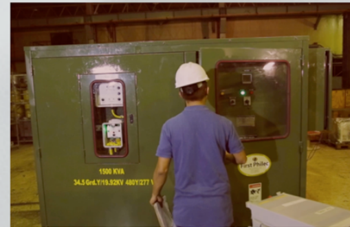
Transformer Preventive Maintenance Services
